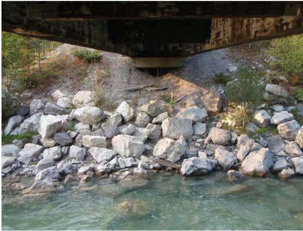
Figure 1-13: Right end abutment.
