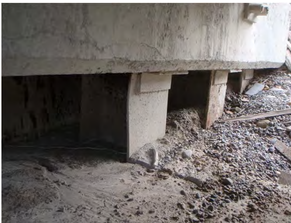
Figure 1-15: Left end abutment piles.
