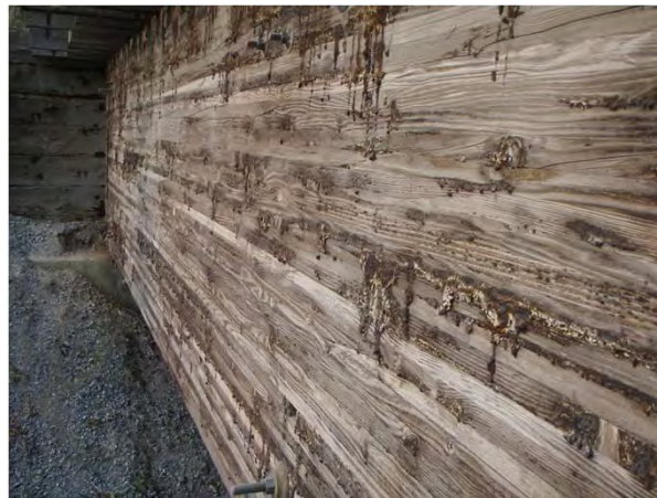
Figure 1-12: Downstream face of span 4 - girder 2.
