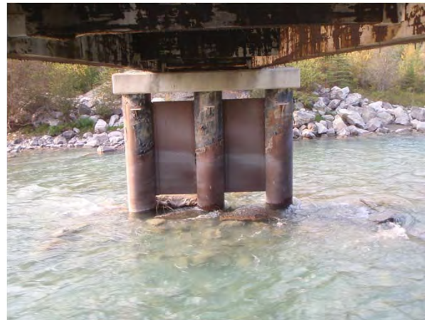
Figure 1-20: Pier 3 from left end.
