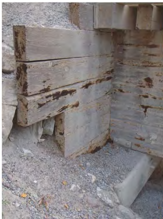
Figure 1-17: Left end ballast wall upstream.
