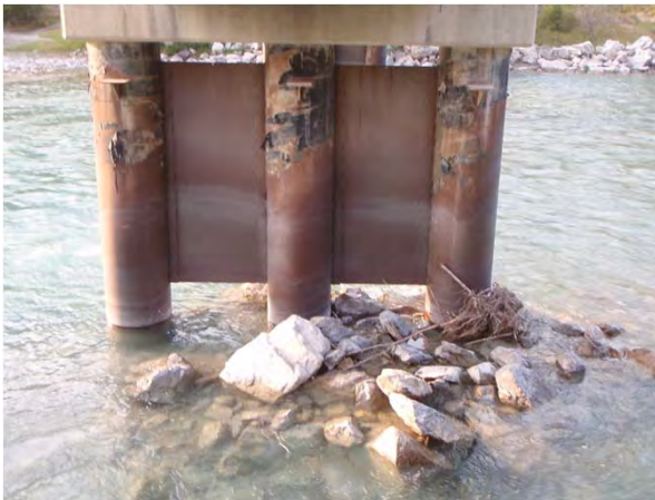
Figure 1-19: Pier 2 from left end.
