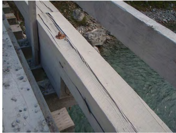
Figure 1-8: Typical curb rail condition.
