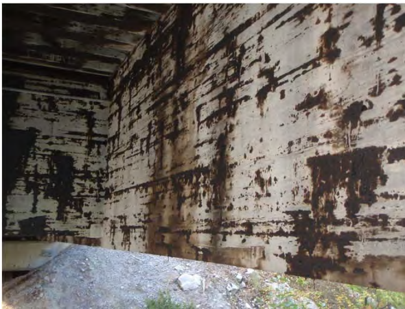
Figure 1-11: Typical interior face of girders.
