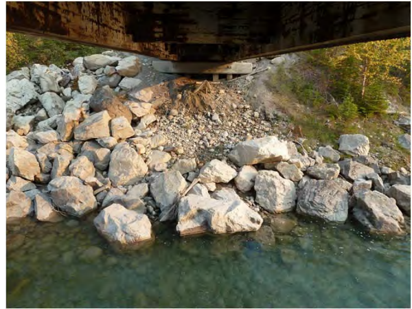
Figure 1-14: Left end abutment.
