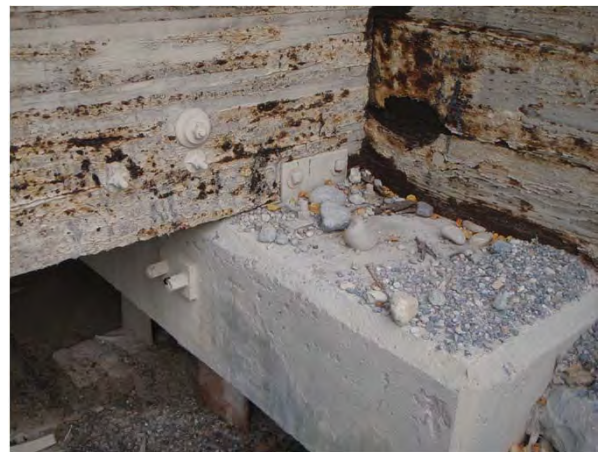
Figure 1-16: Left end downstream bearing.
